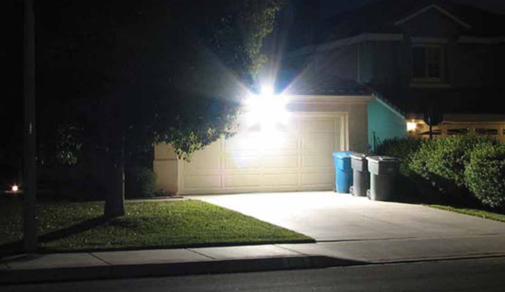
Figure 4: A garage area lit by High power flood light. Flood light distribution, obstruction, results in hard contrast with strong shadows. Such lighting installations will not help to improve security
